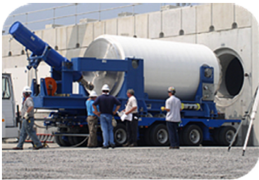
Fig. 5. Loading a canister into a horizontal concrete storage module (Courtesy of Areva TN Inc).
