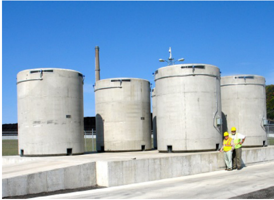
Fig. 4. Vertical concrete casks (Courtesy of NAC International).
